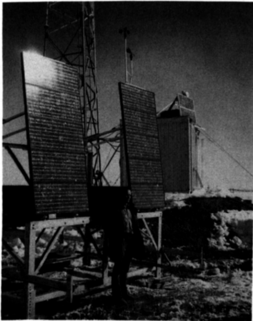
Fig. 1. 80 W/500 A h and 400 W/2000 A h photovoltaic/battery systems installed at Alert (82.5° N), NWT, Canada, and one of the authors (C.L.G.)
